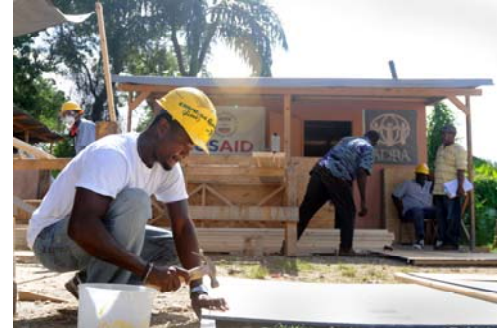
A worker assembles a USAID/OFDA-funded t-shelter. (Kendra Helmer, USAID)
