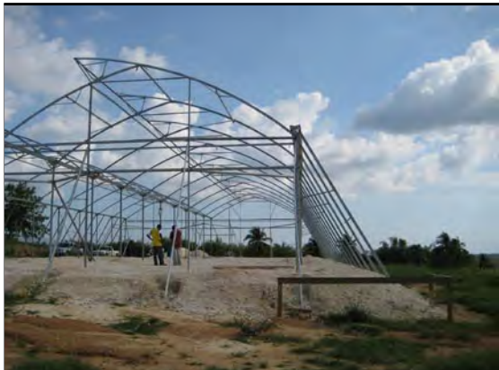
Metal-frame structure being constructed on elevated pad
