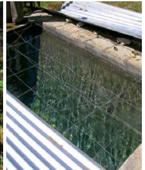
Type: Ferro-Cement Lined Tank Capacity: 6000 and 10000 litres
