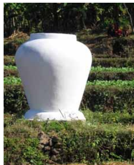
Type: Modified Thai Jar Capacity: 1000, 1500 and 3000 litres
