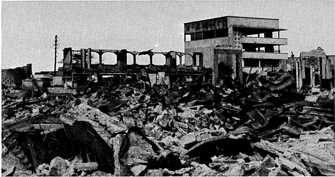
Large areas in downtown Managua lay in ruins as this scene reveals total destruction.
