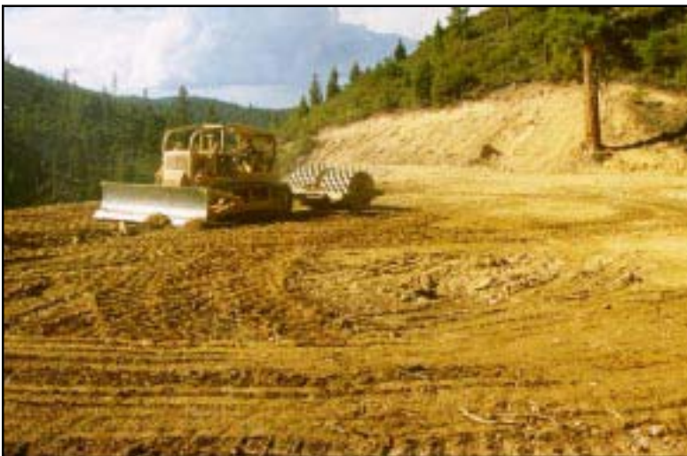
Photo 4.4 Compact the roadway surface and fill material when the road is located near streams or in areas with erosive soils.
