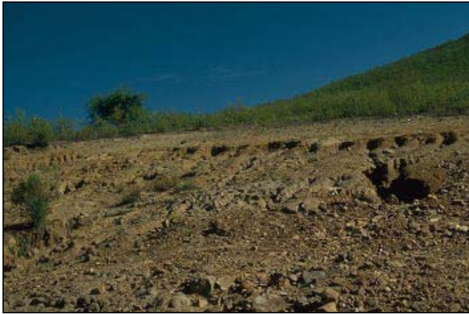
Photo 12.11 This roadside borrow area lacks drainage and erosion control. Roadside quarry development can be inexpensive and useful, but the areas should be hidden if possible, and the areas should be reclaimed once the project is completed.
