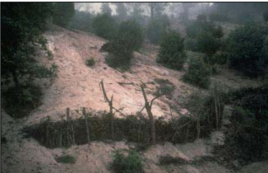
Photo 13.6 Sediment control fences (silt fences), live vegetative barriers, or brush fences can all be used to control sediment movement on slopes (also see Photo 6.6 ).
