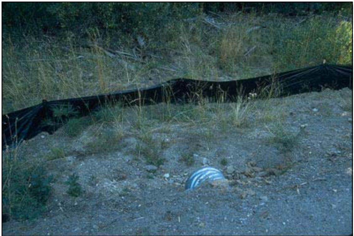
Photo 6.6 Use of a geotextile as a “silt fence” to trap sediment from a construction area.
