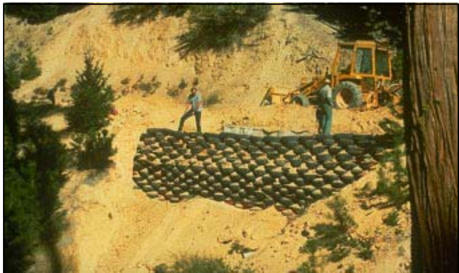
Photo 11.11 A tire-faced, mechanically stabilized earth (MSE) retaining wall, with layers of geotextile reinforcement, being used to gain road width in a fill failure area. MSE (reinforced soil) structures are often the least expensive retaining structure available. Welded wire MSE walls are also commonly used.
