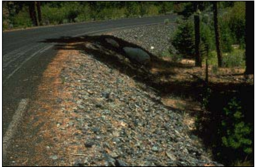
Photo 13.7 Rock armoring, placed on a very erosive soil fill slope adjacent to a creek, used for durable, permanent erosion control.
