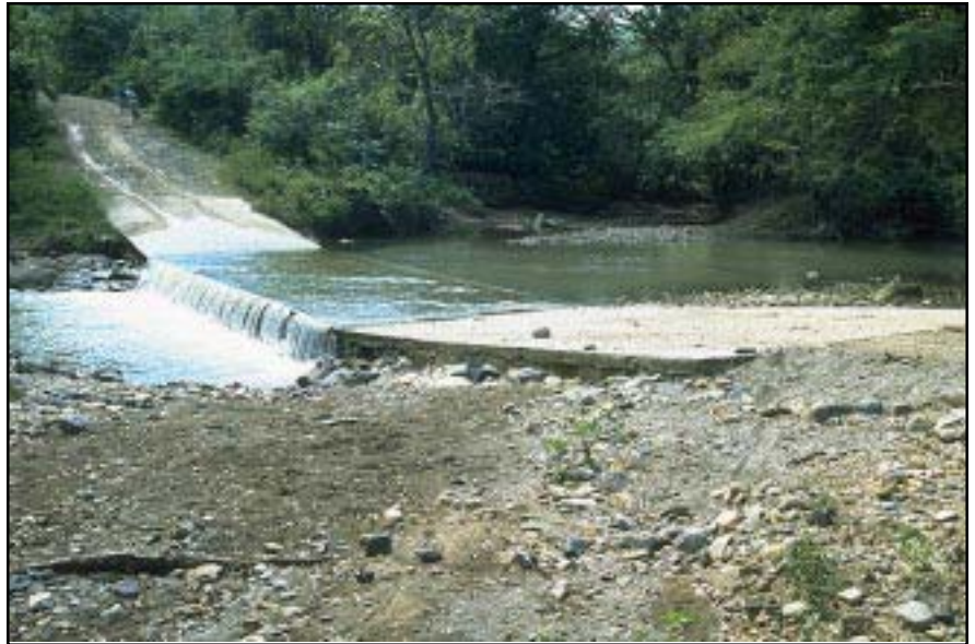
Photo 9.3 With low-water crossings, the downstream edge of the structure typically must be protected against scour and the entire wetted perimeter (to a level above the high water level) should be reinforced.
