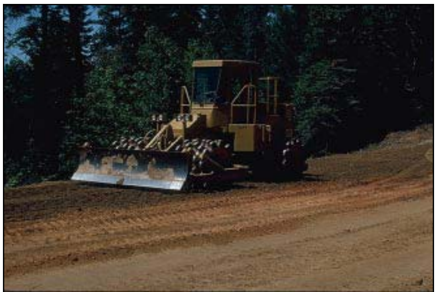
Photo 12.5 Compaction of soil and aggregate is typically the least expensive way to improve the strength and performance of the material. Compaction is useful and cost-effective both for the stability of fill embankments and for the road surface.
