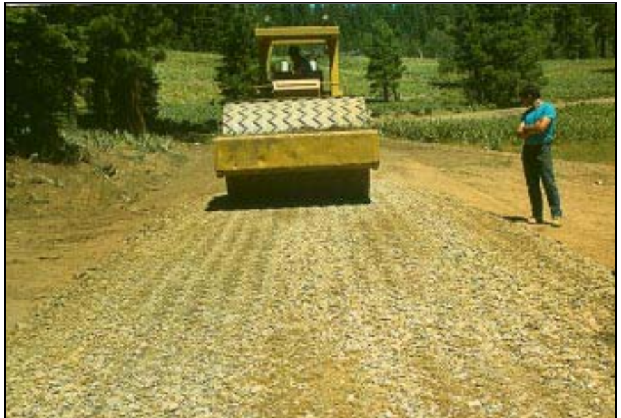
Photo 12.4 A grid roller can be used to produce a desirable surfacing material when the coarse rock is relatively soft. Level and compact the roadway surface aggregate to achieve a dense, smooth, well-drained riding surface.
