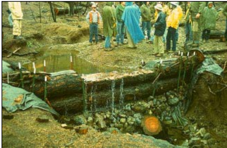
Photo 14.2 Logs being used to build gully stabilization structures in a fire damaged area. Physical or vegetative dams (dikes or debris retention structures) may be used to control sediment and stabilize gullies. Prevent water concentration before gullies form.
