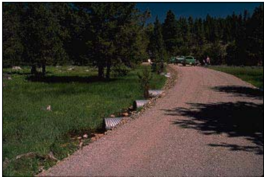
Photo 7.9 Avoid crossing wet meadow areas. When necessary to cross, use multiple drainage pipes to keep water flow dispersed across the meadow.
