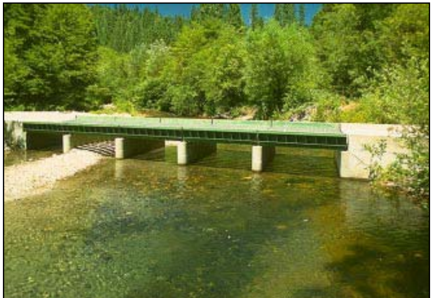
Photo 9.5 Some fords can be designed as “low-water bridge” structures. They must be designed to be occasionally overtopped and have an erosion resistance deck and approaches. This structure is ideal for fish passage.
