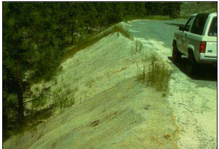
Photo 13.3 Cover fill slopes, work areas, and other exposed soil areas with straw, netting, rock, or other material to protect the ground and promote vegetative growth.
