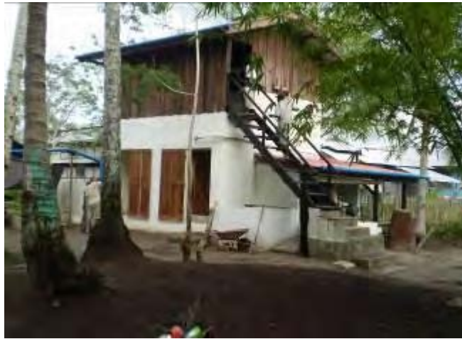
The newly established cool storage site
