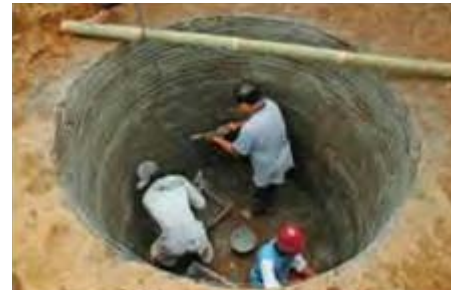
Construction training of rain catchment tanks
