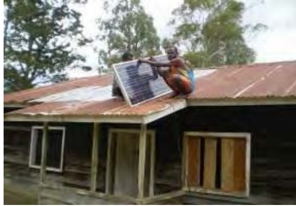
Solar cell installation at Pireme
