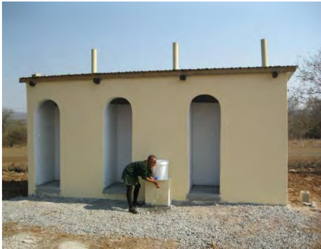
Picture 18. Latrines Constructed in Hluti Central
