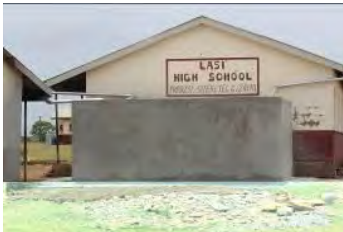
Picture 16. 75m 3 RC tank in Ngcina/Lasi High school, Mpolonjeni Inkhundla
