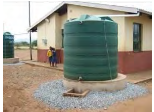
Picture 15. Upgraded RWH system at Phumelela Primary School Matsanjeni Tinkhundla
