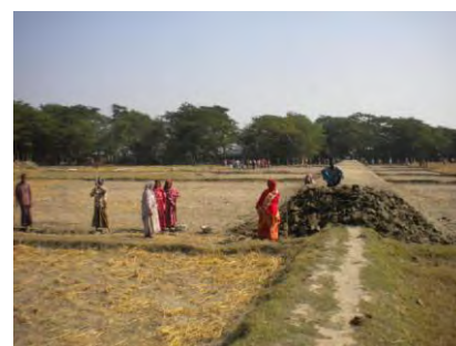
A raised road cum dykes under construction
