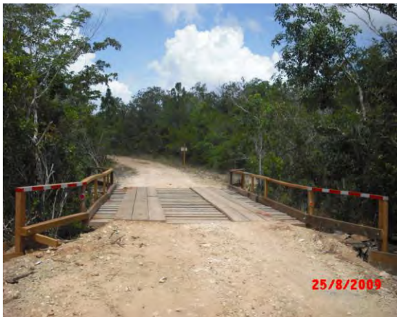
(One of the five bridges repaired – Tiger Creek)
