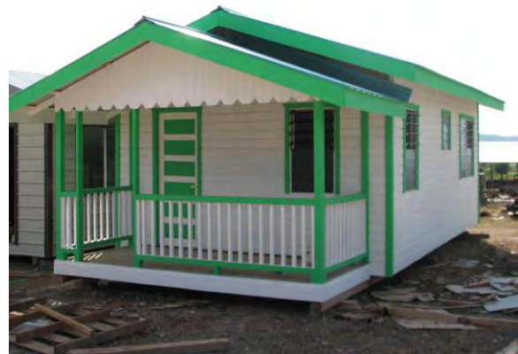
(New Guard house at East Gate access point)
