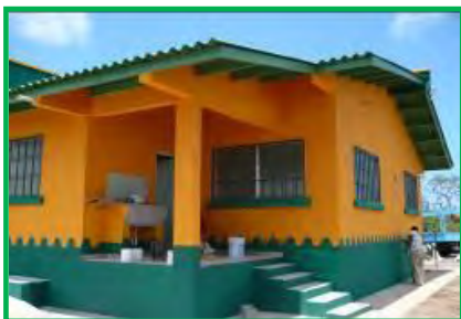
New park sub-station in Cuango community.
