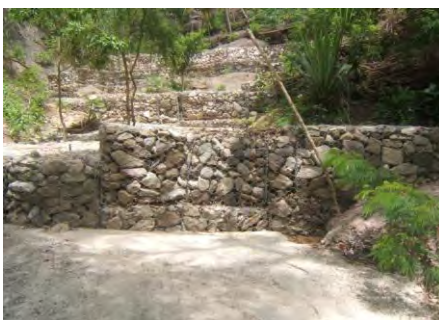
Project site after
