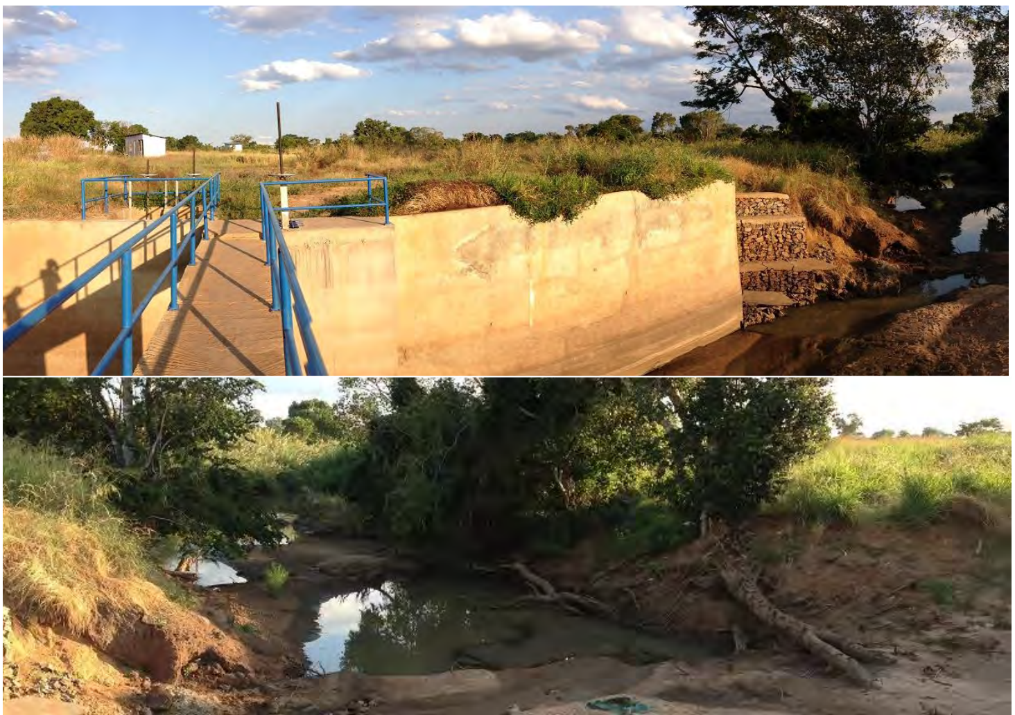
Figure 28: (Top) Irrigation intake at Lukenge, where water level marks can be painted on the wall for monitoring water level (Bottom) The Mkindo River in the dry season at Lukenge. The river rises 4 m higher in the wet season as evident from the incised channel and from local anecdotes
