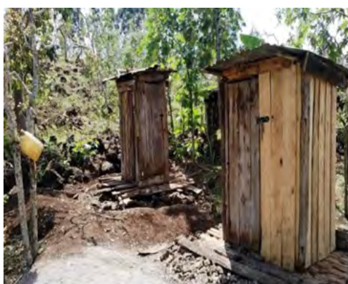
Latrines constructed after community IPC orientations
