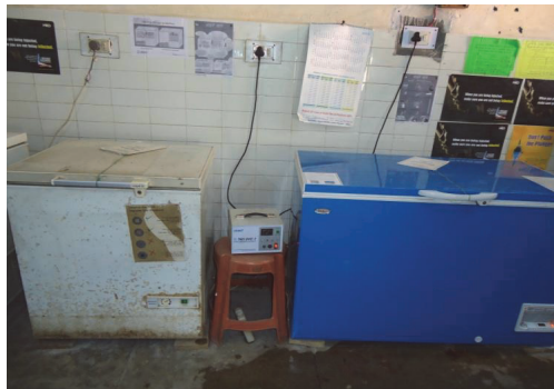
Preventive Maintenance of Cold Chain Equipment Before (Left) and After the Intervention (Right)
