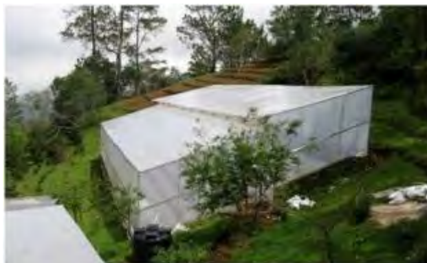
Mevs greenhouse with open top for ventilation
