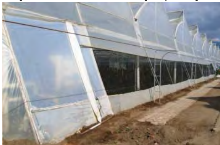
Ecuadorian greenhouse with side and top ventilation.
