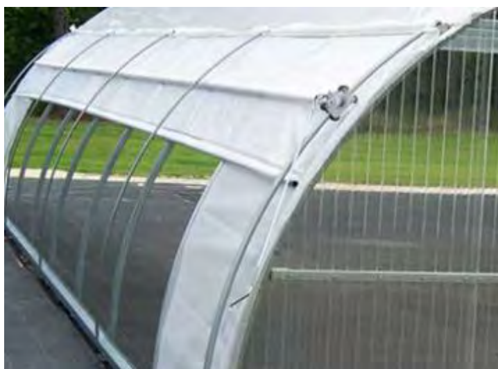
Example of simple roll up mechanism on hoop house.
