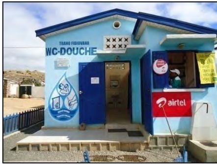
This public WASH block in Ambanitsena is located 20 km from the capital.
