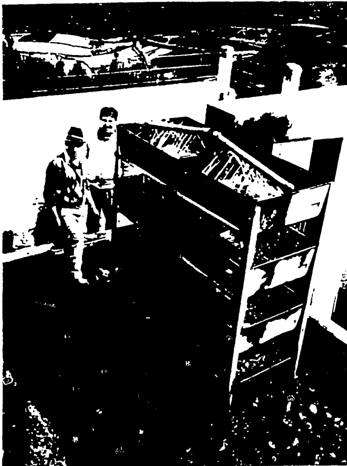
PHOTO NO. 14: This aerator is part of the water treatment plant in the community of Llimpe, in the province of Tungurahua. The aerator is needed as part of a treatment system which removes an excessive concentration of iron from the water. The treatment plant is sophisticated, with aeration, sedimentation, slow sand filtration, and chlorination. O&M is surprisingly good, with the only part of the system which is not adequately operated and maintained being the chlorination facility, because there is a lack of funds to pay for chlorine, and therefore the chlorination is intermittent.
