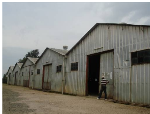
Abandoned and unused former strategic grain storage facility
