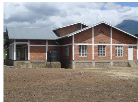
New seed potato storage facility
