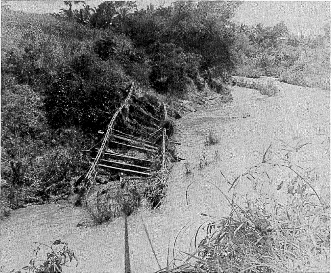
A bridge destroyed by flood waters in Capiz Province.
