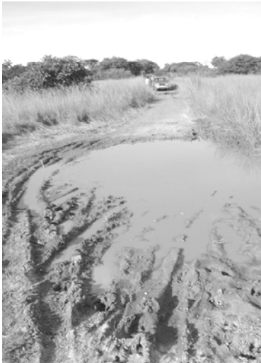
A rural road in Zambia. Upgrading the road will require elevating the roadbed across a wetland area, adversely affecting local water flow. Could USAID funds still be used for this project?
