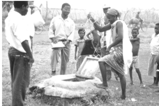
A low cost alternative to a hand pump—a privately owned shallow well with a trap door cover near Segou, Mali. Note that water retrieved may require treatment to achieve desired quality according to end use.
