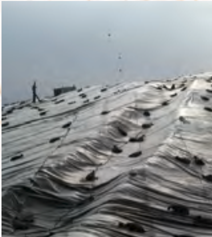
Sandbags holding down final cover.
