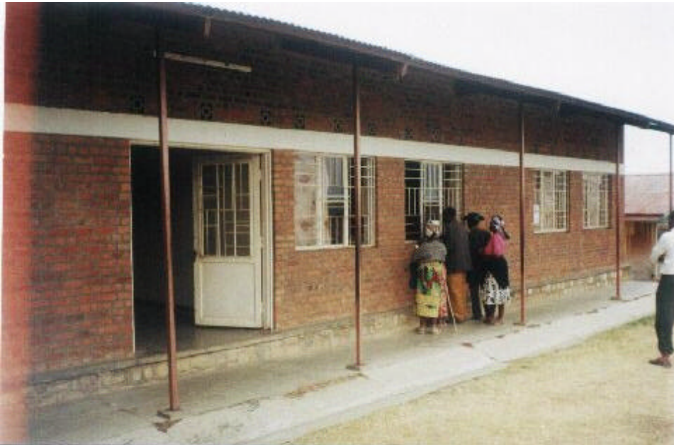
Mabanza Canton Court --In order to talk to the court clerk, litigants must speak through the window.
