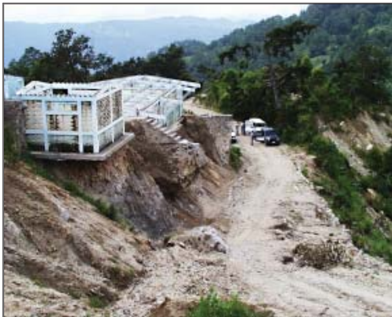
Figure 6. View of the El Pinar landslide and the abandoned school. A new road has been graded across the head of the landslide, which slid into the valley of the Río La Palma o Las Pozos on the right. Future movements on the landslide will likely disrupt the new road.
