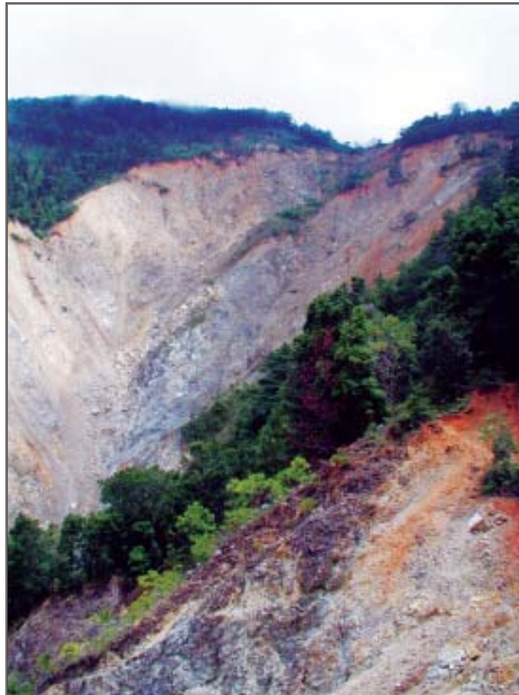
Figure 5. View to the northeast of the upper part of El Zompopera landslide. The collapse of unstable blocks in the upper part of the landslide destroyed a road at the crest of the ridge. Many unstable blocks remain in the upper part of the slide and a catastrophic collapse of those blocks could potentially dam the Río La Palma at the bottom of the valley.
