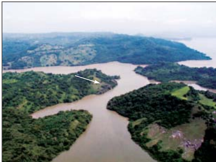
Figure 17. Shallow landslide on the shore of Embalse 15 de Septiembre. The scar was largely vegetated when this photograph was taken in September 2001.
