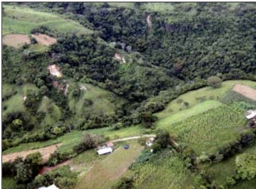
Figure 12. Scars of landslides caused by the 13 February 2001 earthquake west of San Lorenzo. Like the Hurricane Mitch landslides, these shallow landslides caused little serious damage, but repeated sliding here shows that these slopes are highly susceptible to landslides.
