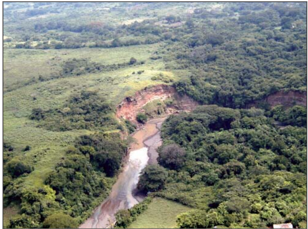
Figure 18. Bank failure on the Río Gualcho about 4 km upstream of Embalse 15 de Septiembre. This and similar failures along the Río Gualcho may have resulted from accelerated bank erosion cause by the high stream flows that occurred during Hurricane Mitch.
