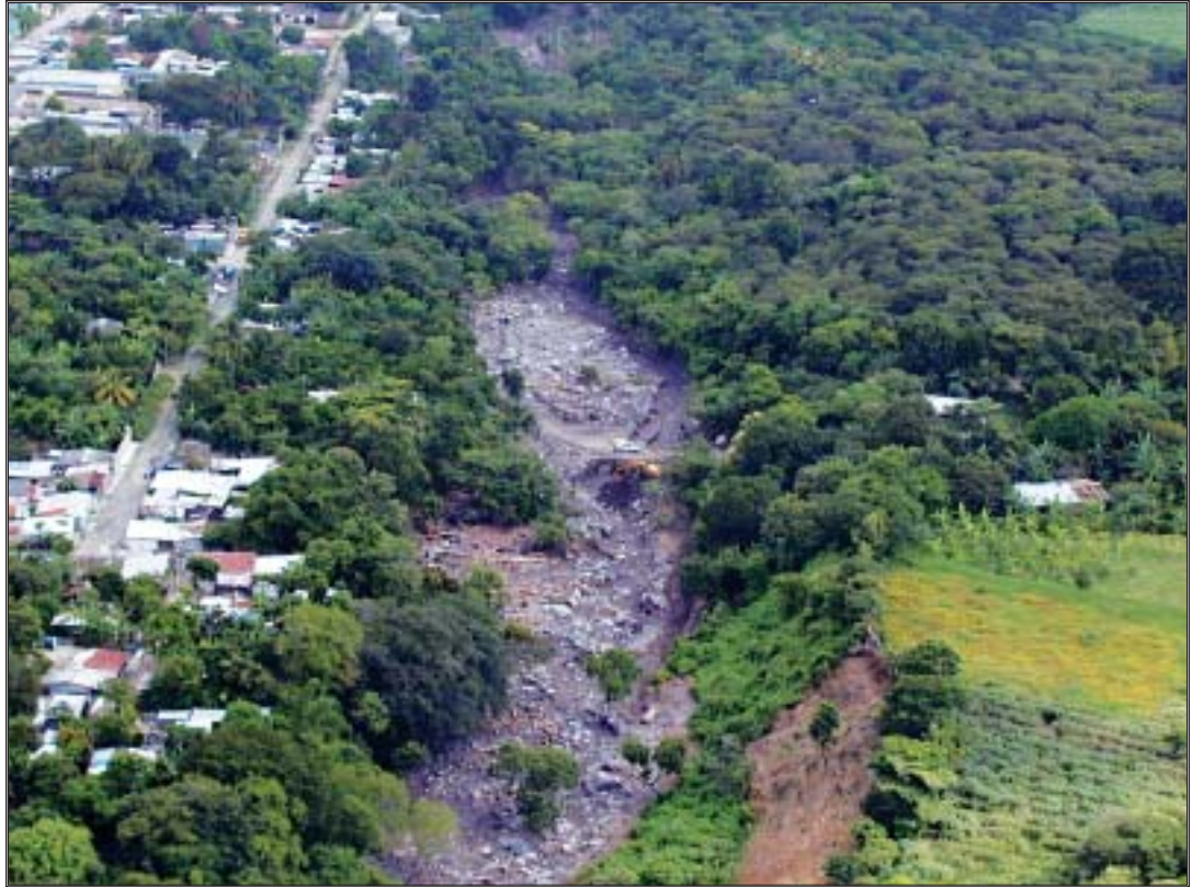
Figure 10. Oblique aerial view of the debris flow on the northeast side of the town of Guadalupe that occurred on 15 September 2001. Many of the large boulders in the channel were transported by the debris flow.
