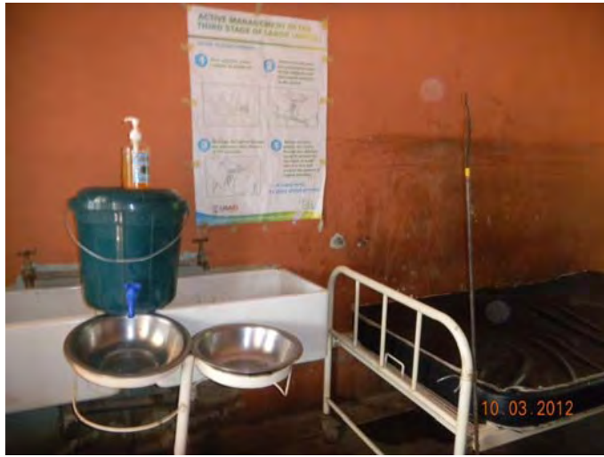
Photo 3. Lack of hygiene in delivery rooms.
