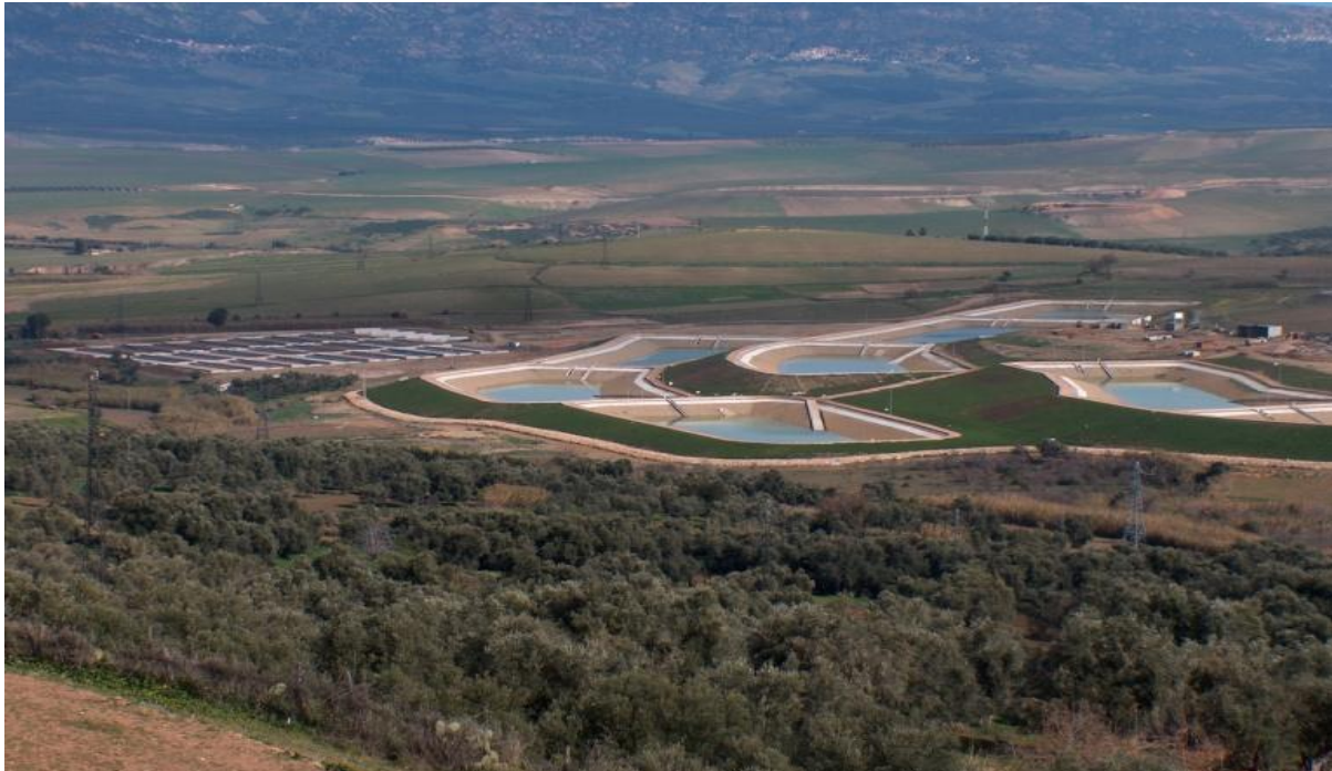
Meknès wastewater treatment plant
