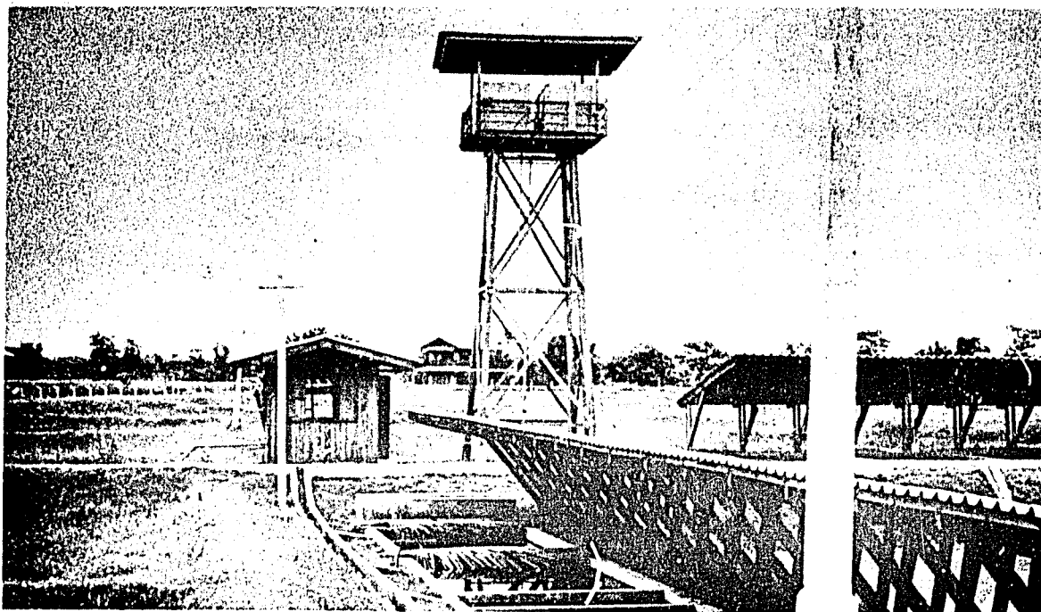
Fig. 3. Concrete-lined water supply canals are used at Maha Sarakham and Khon Kaen. Overhead tanks are used to supply small ponds or concrete pools constructed above soil level.
