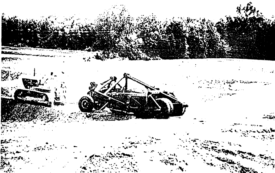
Construction of experimental ponds is a continuing program at Auburn.
