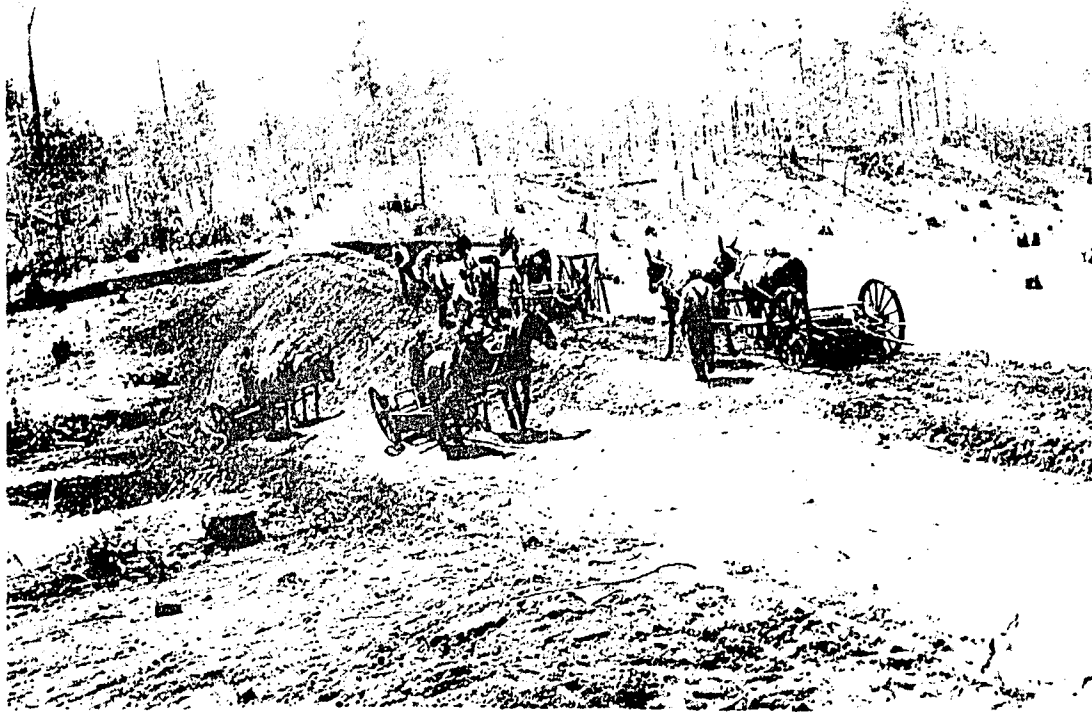
The first ponds at Auburn University were constructed in the early 1930's with mules, scrapes and much manual labor.
