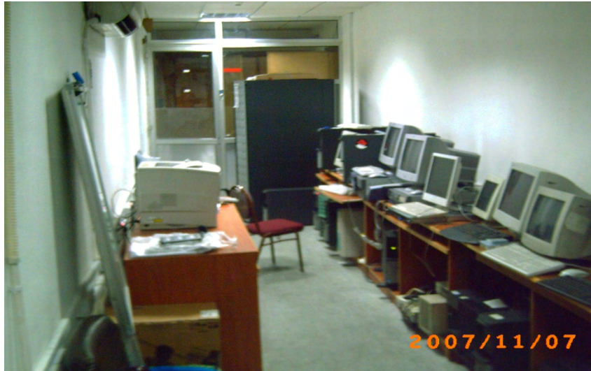
Jordan Customs' data center prior to Program technical assistance.
