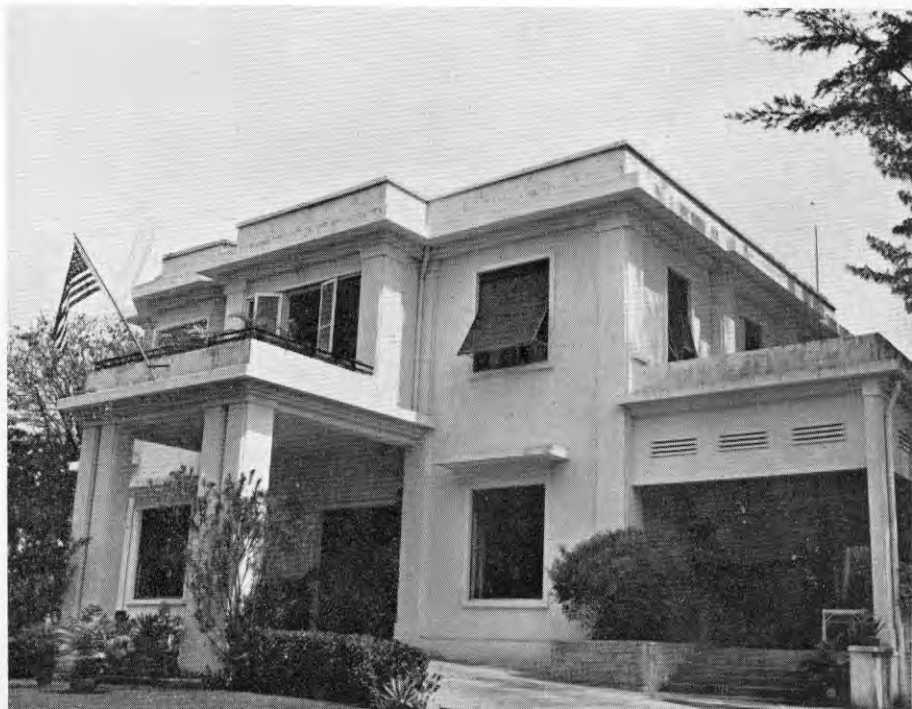
The American Embassy residence
