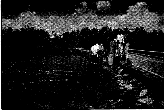
Causeway impeding the flow of lagoon water will be replaced by a bridge
