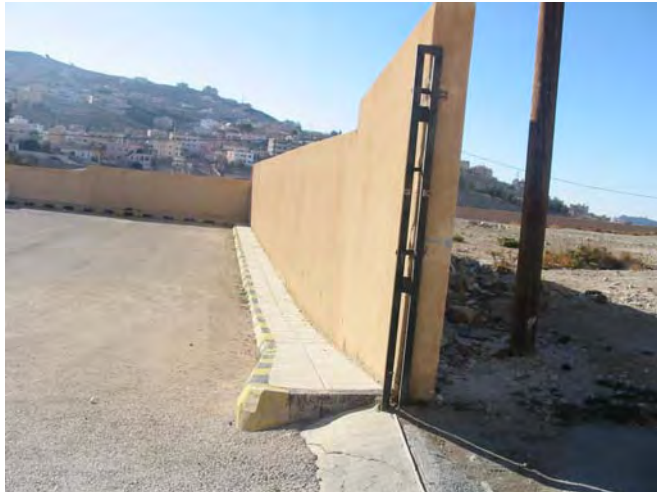
Figure 1.9: Wall Separating the Land Plot from the Adjacent Sport Center
