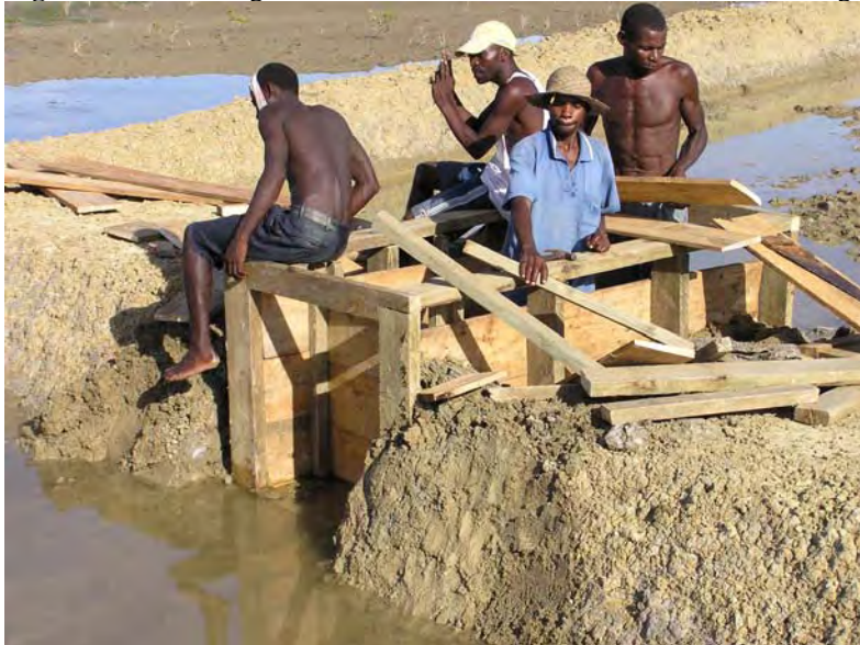
Figure 16: Wooden gate under construction at Mkadam farm, Mkuranga, Tanzania
