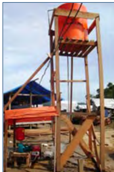
Figure 3-3 Well Installation in Calang – 2005.
