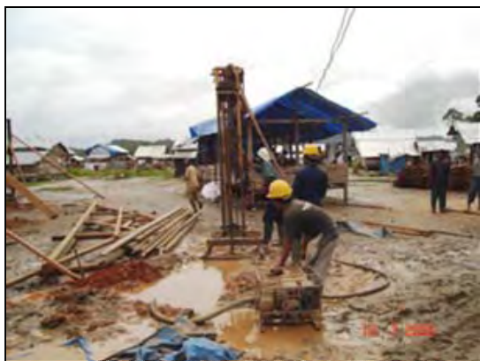
Figure 4: Drilling of Well at Lhok Buya near Calang (IRC photograph).
