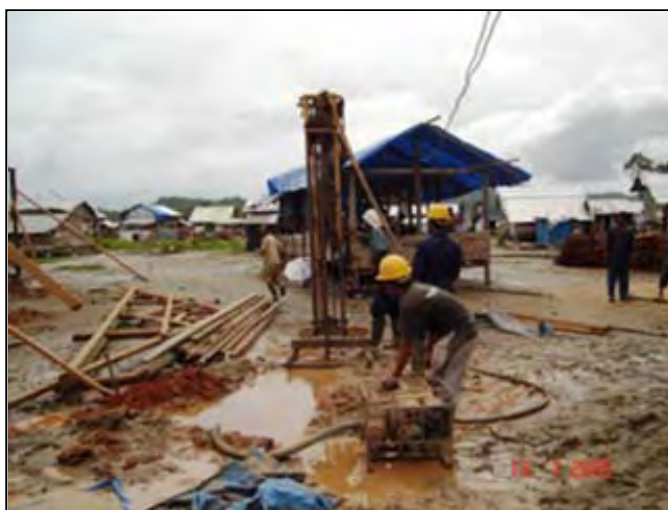
Figure 5: Well Drilling in Aceh.
