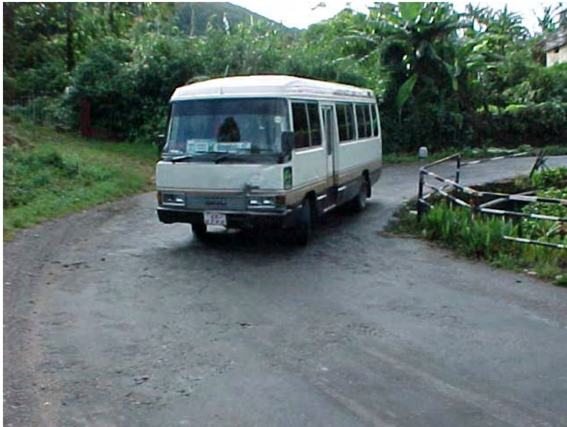
Figure 5-6. Typical Turn and Culvert on Highway 7
