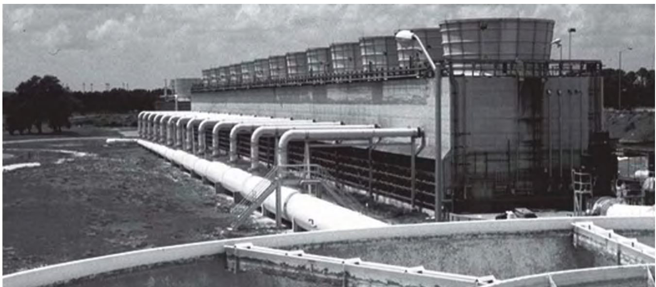
Figure 2-3. Cooling Tower
