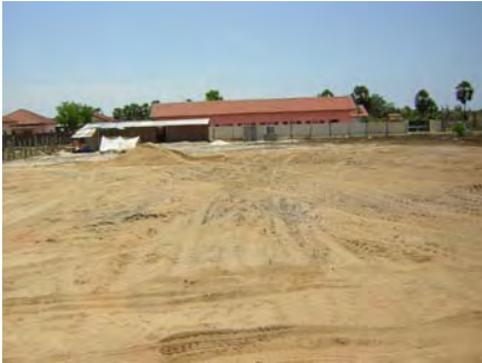
Figure 19- Photographs of the Kaluwanchikudi site
