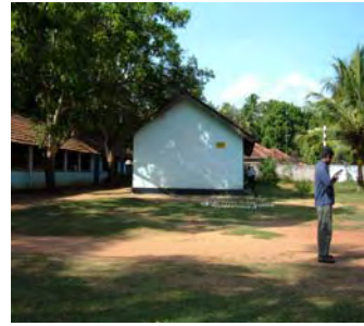
b) View of the existing VTC buildings
