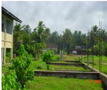
b) A closer view of the foundations of the destroyed building
