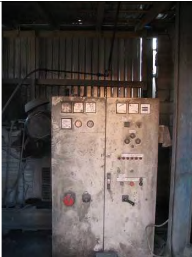
Control system for heating
