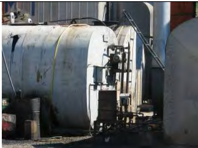
Bitumen and fuel storage
