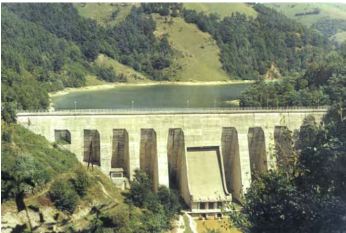
Secu Dam and Lake – r. Bârzava
