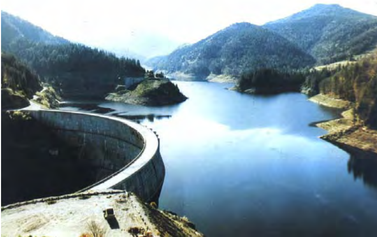
Drăgan Dam and Lake – v. Drăgan (b.h. Crișul Repede)
