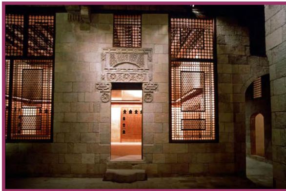
Al-Hawari House restoration, 18th century Ottoman house, Cairo Egypt
