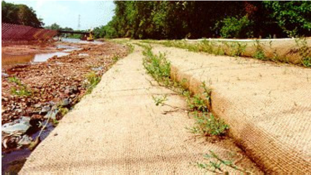
Figure 24. Coir blankets used for river bank stabilization.
