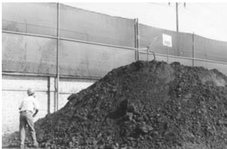
Figure 9. Moistening and new fences at the CENTROMIN storage facility, May 2000. Courtesy of Jose Luis Quequejuna.
