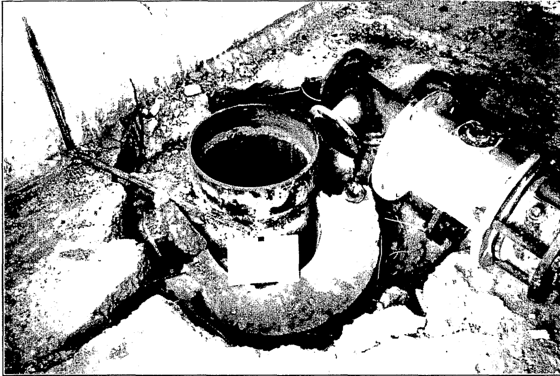
Photo 8. Well 30 showing collapsed floor surrounding well casing.
