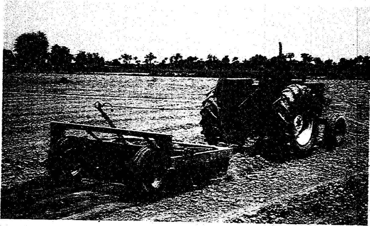
Figure 4.12. Levelling construction with trailing scraper.
