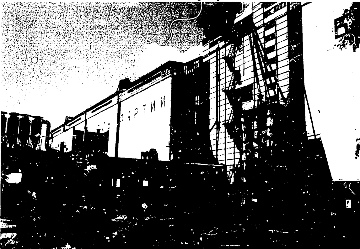
State Elevator, Pre-Cast Construction
