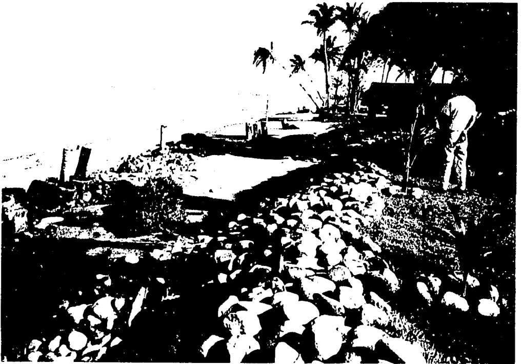
Plate 4. Revetments protect this beach resort in Langayen Gulf, Philippines.
