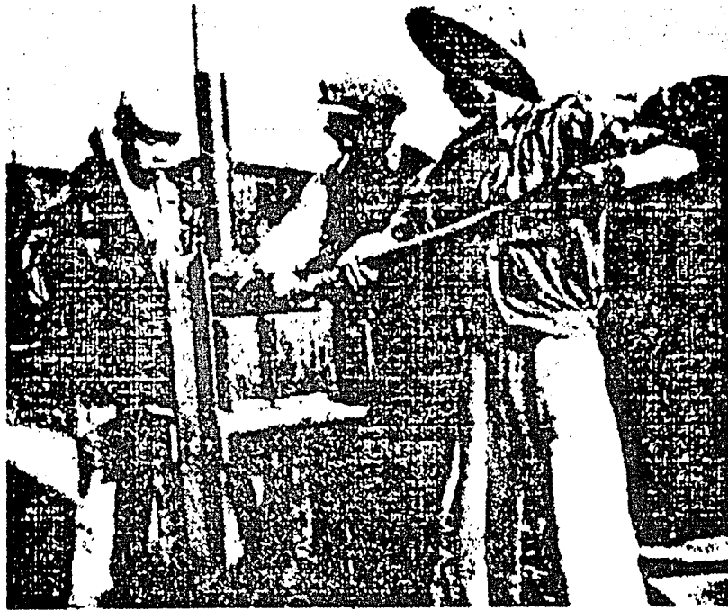
The Dampened Earth Mixture is Placed in a Machine to Form Building Blocks Under Pressure.
