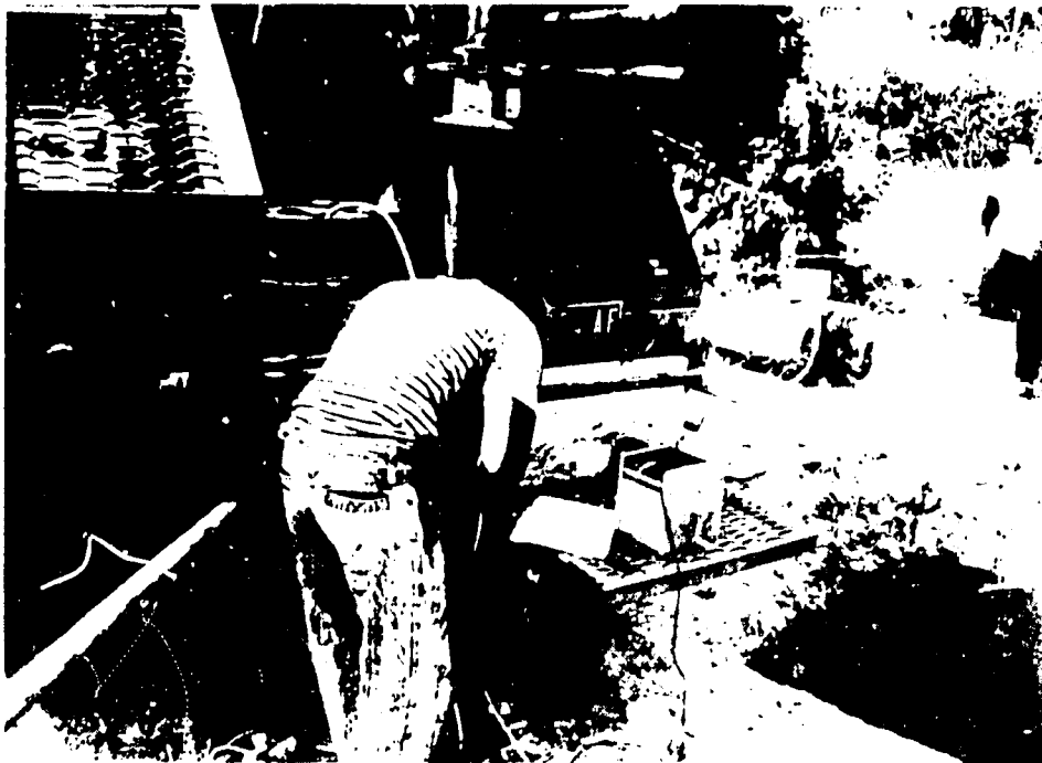
7. Taking borehole pumping level readings at Amapu
