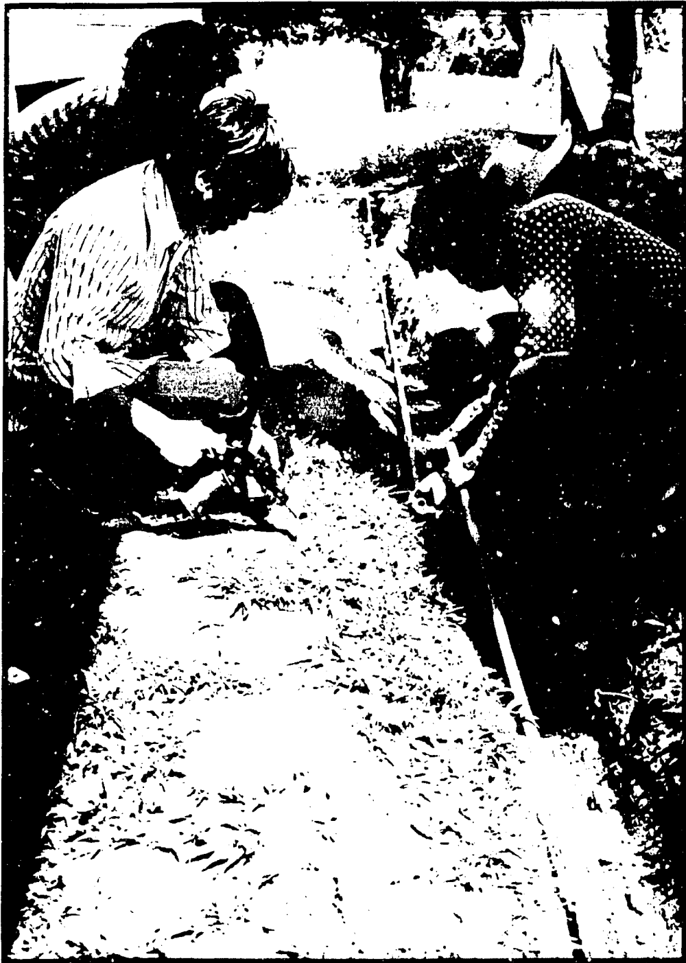
Illus. 12. A gravity system being installed. (Source: WHO, Photo by J. Abcede.)
