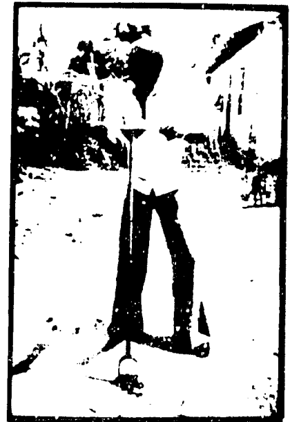
Illus. 17. A hand augured well. (Source: Blankwaardt. Hand Drilled Wells: A Manual on Siting, Design, Construction and Maintenance . Rwegarulila Water Resources Institute, Dar Es Salaam, Tanzania, 1984.)
