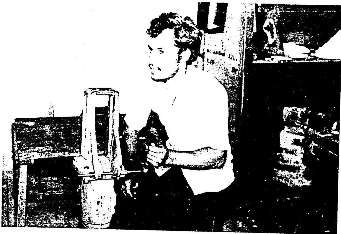
CAP REAMING TO CORRECT MISALINGED DRILLED HOLES
