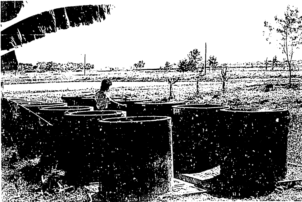
Circular concrete tanks at the Bureau of Fisheries and Aquatic Resources National Freshwater Fisheries Technology Research Center, Muñoz, Nueva Ecija, Philippines, built for the project's on-station growth trials with different strains of Oreochromis niloticus .
